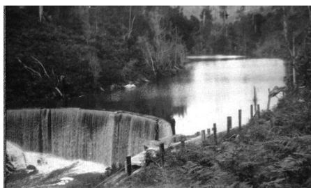
The full weir
