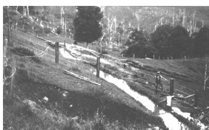
Head race to Tunnel
