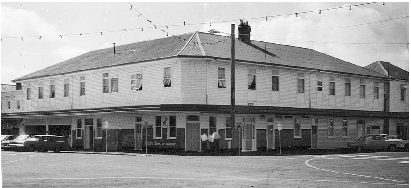
Rebuild completed with installation of cantilevered awnings 1971
