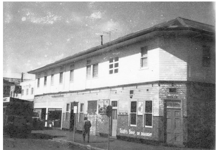
Court House Hotel looking sad 1971
