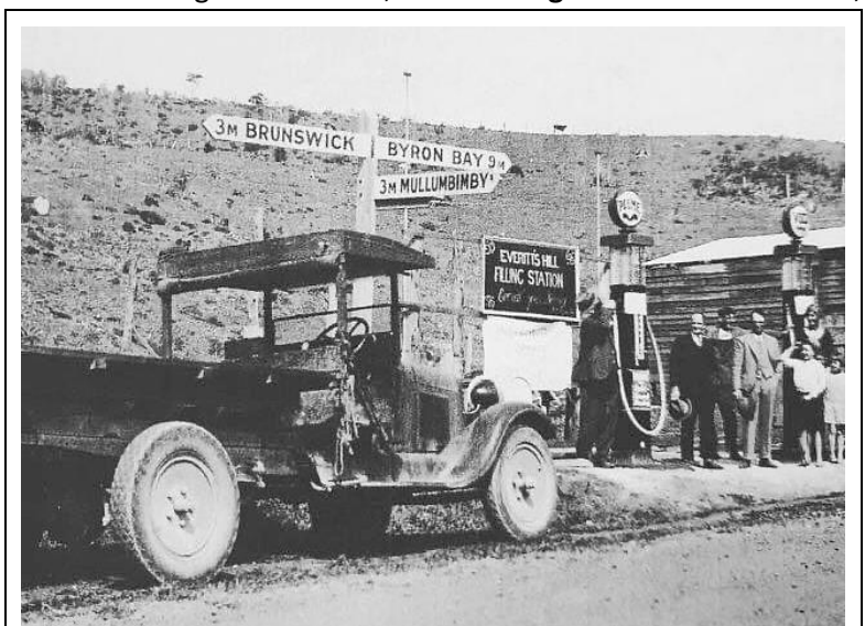
'Everitt's Hill Filling Station'
