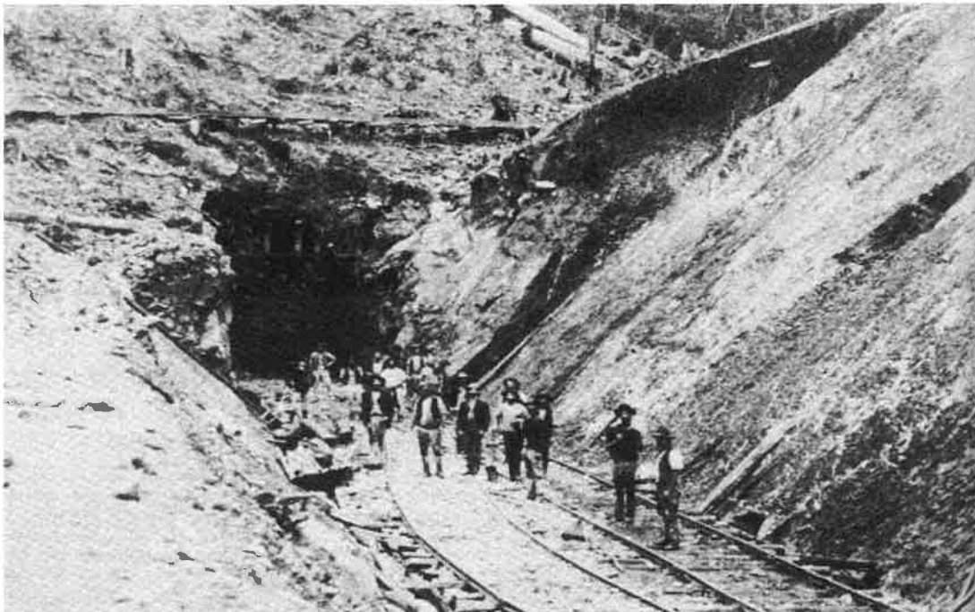
Lismore to Tweed Railway Tunnel
